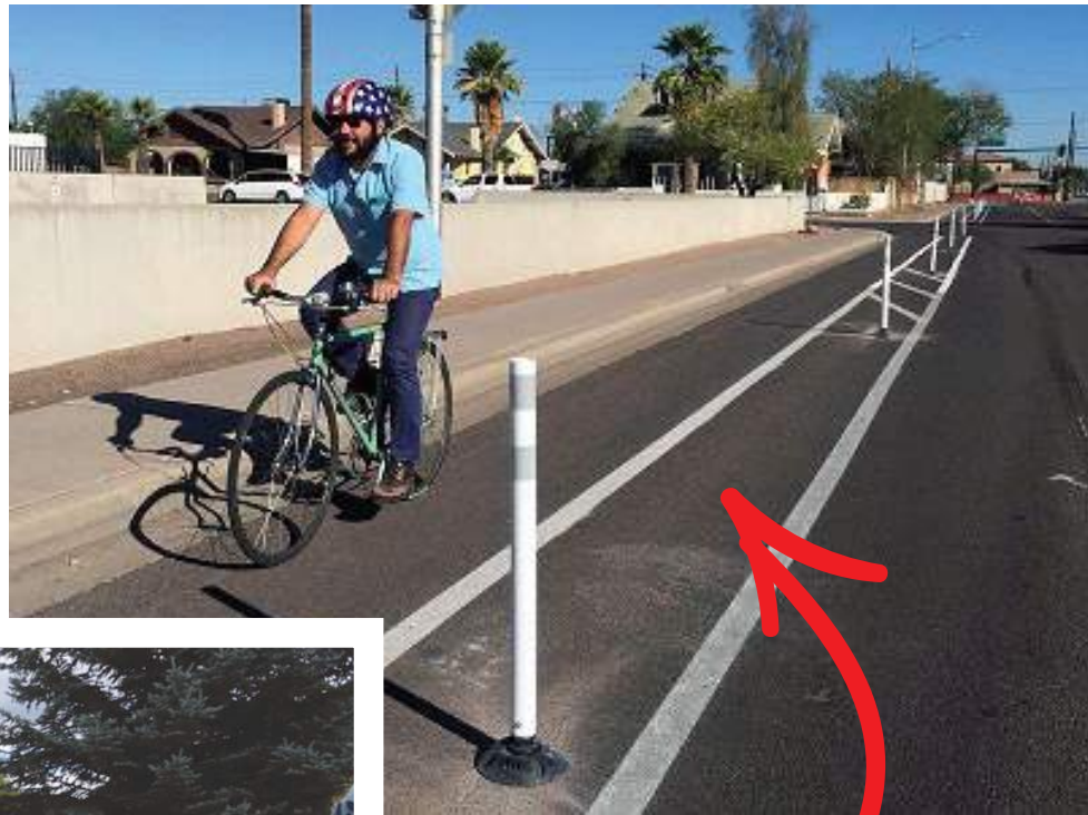
Bollard-protected bike lane (Short Term and Low-Cost Improvement)
